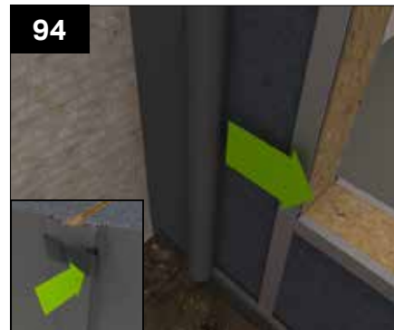
94 Unroll the membrane over the walls allowing this to sit slightly below DPC level (around 10 mm). Ensure that any joins in the membrane overlap by a minimum of 100mm horizontally and 150mm vertically. This can be clipped in place using the membrane clips provided. The membrane detail at the top of the wall is shown in the following steps.
