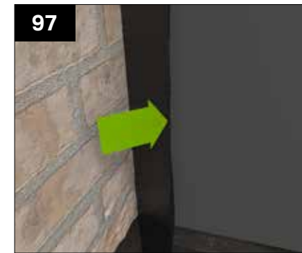
97 At the host wall fold the vertical DPC over the top of the membrane prior to battening out.
