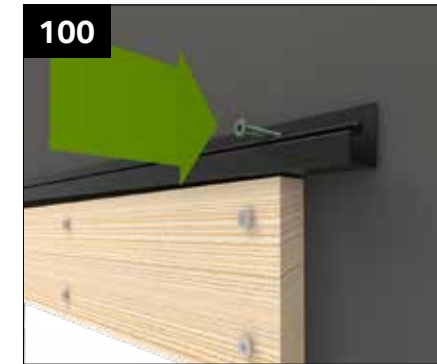
100 Fit the soaker trim to the wall at a slight angle using the GPHS fixing at 450mm centres, giving it a roughly one-degree fall. The battens should terminate above and below this trim.
