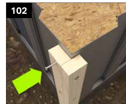
102 At corners battens should be fixed as shown. This ensures that wall finishes (claddings) at the corners are well reinforced.
