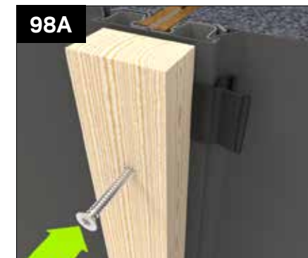
98A Position a 25mm batten, treated timber (optionally provided) or alternative, against the clips trapping the membrane in place. At apertures this batten is positioned inline with the opening as shown in image B. Secure the batten to the walling full and half clips at 450mm centres using the winged fixing screw (provided with battens). Please Note: - Excluding Flat Roof, the battens will be shorter than the clip length and should be set down from the eaves level or other air flow obstructing roof elements by 12mm to allow for ventilation.
